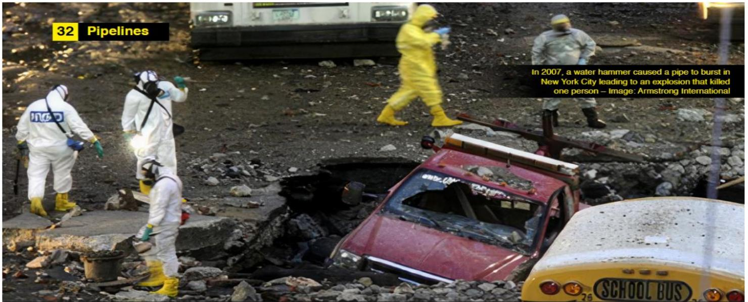
In 2007, a water hammer caused a pipe to burst in New York City leading to an explosion that killed one person – Image: Armstrong International
